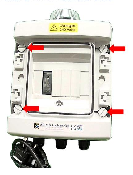
Fasten the lid to the enclosure using the 4 plastic screws.
