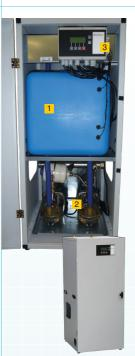
The 75H is a complete rainwater system with integral storage tank [1], dual pump pressure raising unit [2] and electronic controller [3].
